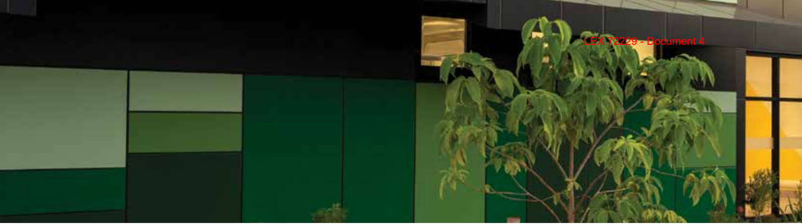
Above: Berrimah Farm Science Precinct new Molecular Diagnostic Science Laboratories - Credit: Department of Infrastructure, Planning and Logistics.
