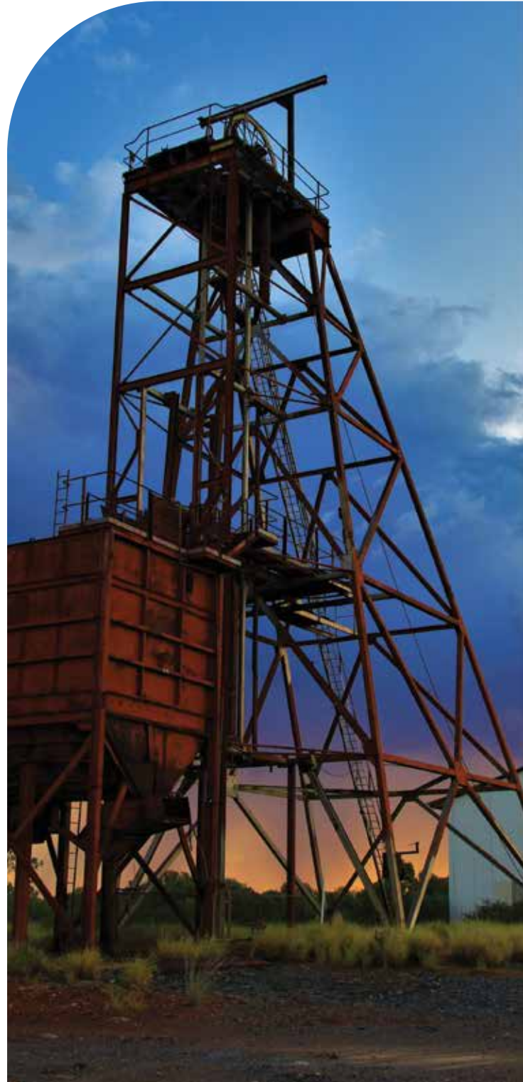
Above: Gold mining infrastructure Tennant Creek. Credit: Efsta Konidaris.
