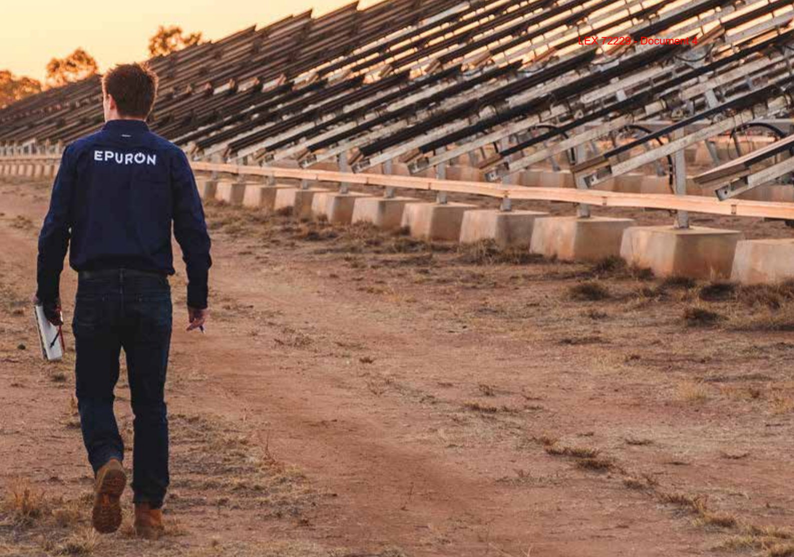
Above: Katherine Solar Farm. Credit: Department of Industry, Tourism and Trade / Investment Territory.
