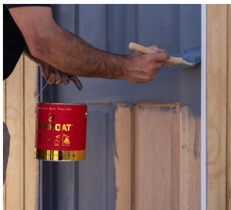
FIRECOAT external paint developed for extreme fire protection (left), FIRECOAT fire suppression and protection paint test (right)
