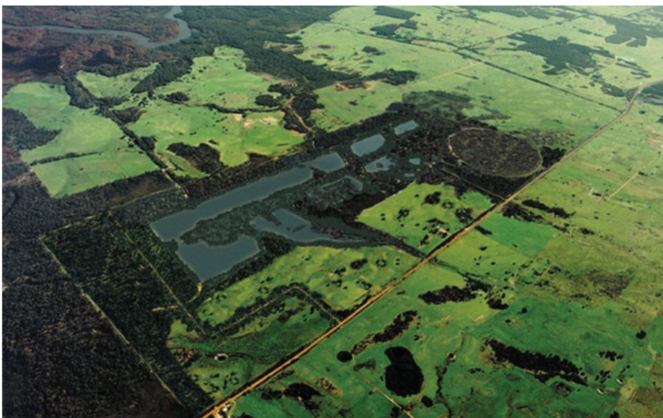
Figure 5.8 - Beenup mine, 3 years after closure
