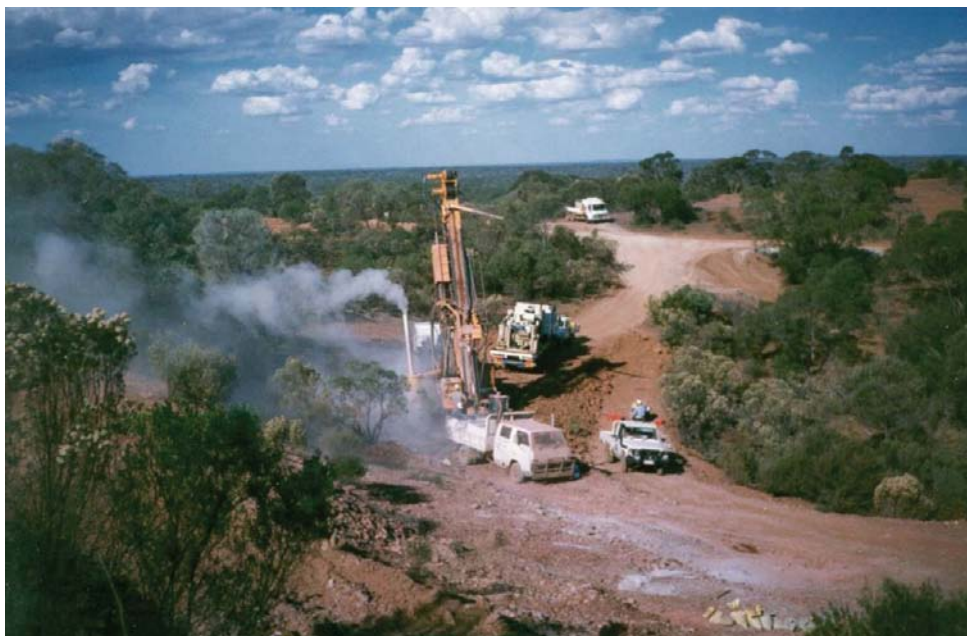
Figure 2.1 – Exploration drilling can produce significant sustainability impacts (photo - Roberts - DMR - http://www.mining.unsw.edu.au/kcmi/Govern/NSW_DMR_2.pdf )
