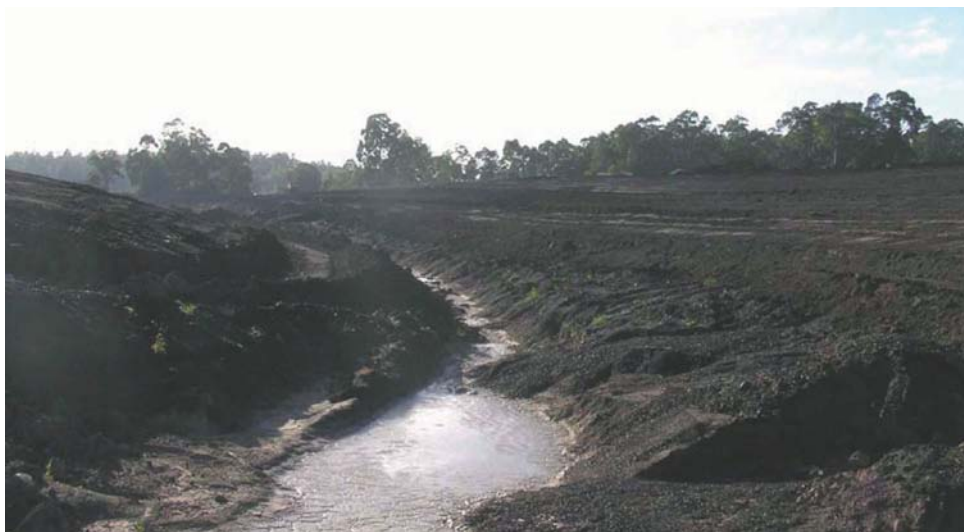
Figure 5.38 - Re-establishment of Maryland Creek, New Wallsend mine
