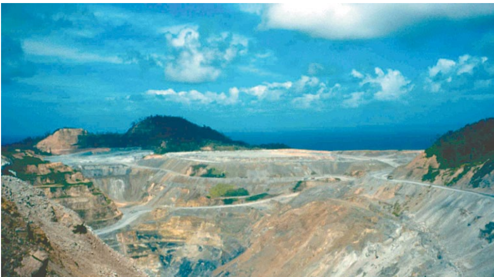
Figure 5.12 - Misima before rehabilitation
