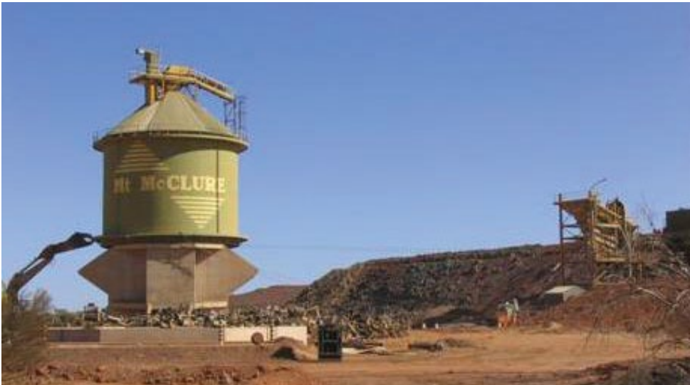
Figure 5.10 - The Mt McClure site before closure
