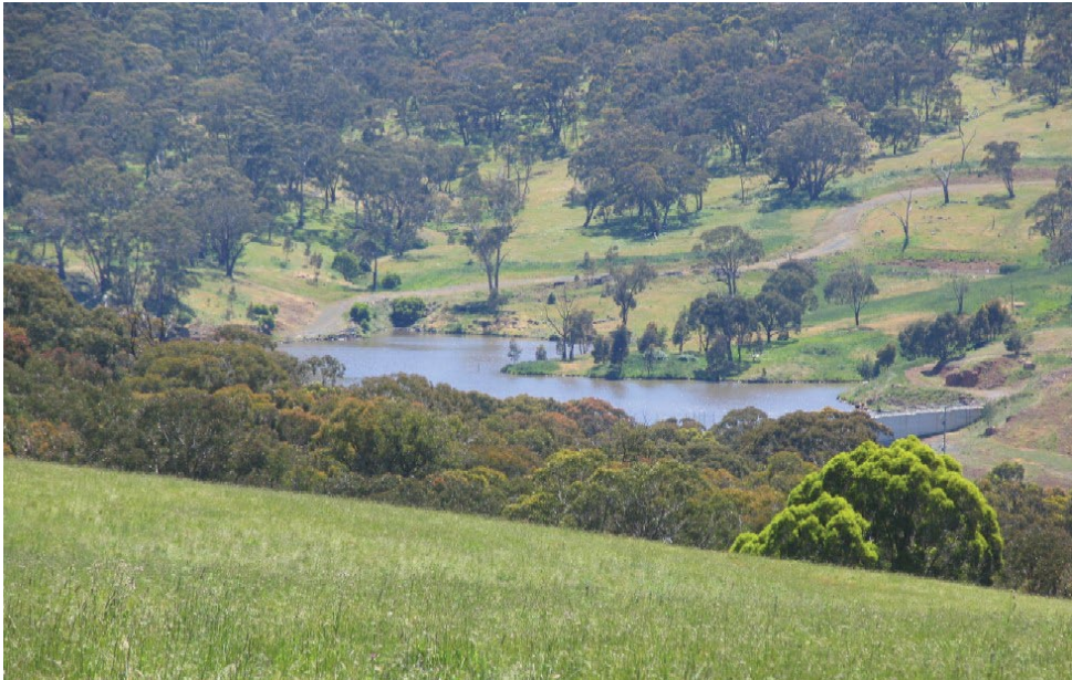
Figure 2.16 - Cadiangullong Creek Dam
