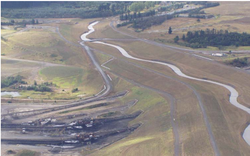
Figure 3.6 - Construction of the Morwell River diversion
