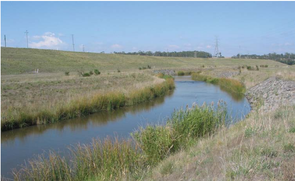
Figure 3.7 - Morwell River after diversion
