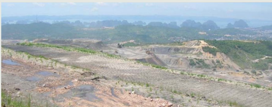
Figure 4.16 - View over Ha Long Bay from top of waste dump
