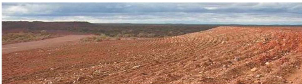
Figure 5.26 - Concave waste dump slope at Murrin Murrin
