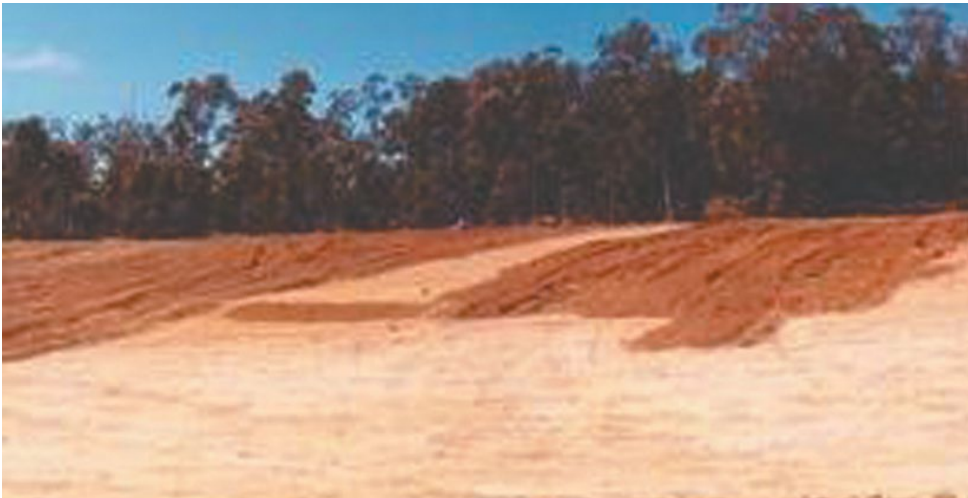
Figure 5.29 - Spreading topsoil at an Alcoa operation
