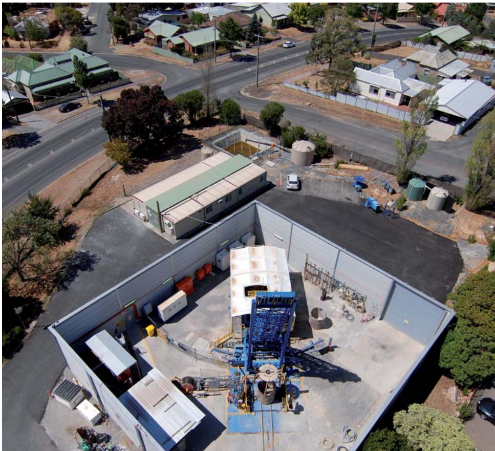
Figure 3.2 - View of the worksite showing proximity of residents
