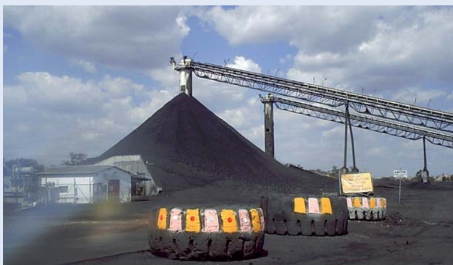
Dump station showing the effect of coal stockpiles. Source: Emma Charlton, AECOM.
