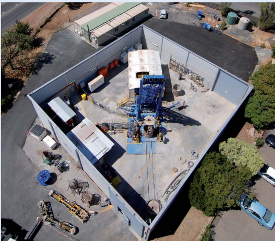
Bird's-eye view of the worksite in Ballarat. Source: LGL - Ballarat Goldfields.
