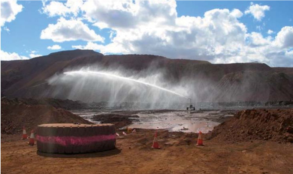
The mobile irrigator being used to wet the iron ore in the pit. The direction of travel is towards the anchor. A rotameter driven by the water winds the cable up onto the cable reel. Source: John Visser, Rio Tinto.
