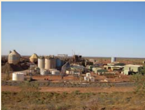
Granites processing facility
