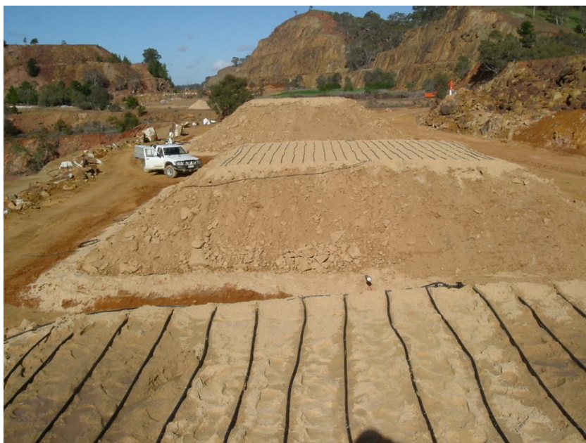
Figure 17: Test pads constructed at the Brukunga legacy site in South Australia
