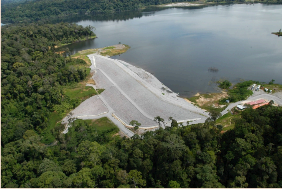
Figure 2: Namuk tailings storage area showing constructed embankment
