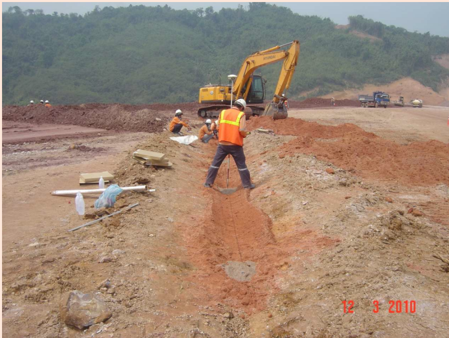
Figure 4: Installation of horizontal pore gas monitoring system
