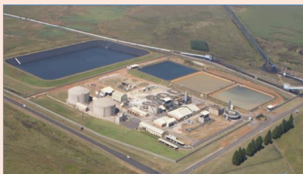
Figure 1: Phase 1 of the water reclamation plant
