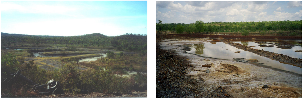
Figure 30: Wetland constructed to polish seepage from a covered WRD, during initial years of neutral drainage (left), and after it was overwhelmed and rendered ineffective by breakthrough of highly acidic and metal-rich seepage (right).
