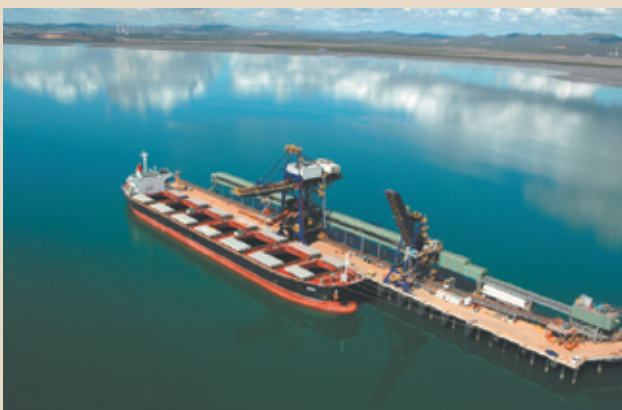
Bauxite shipment to Alumina Refinery (Rio Tinto Aluminium Limited), Gladstone, Queensland
