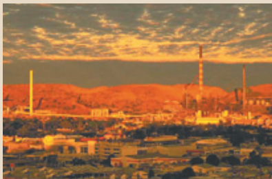
Xstrata copper smelter at Mount Isa Mines—copper smelter (red and white stack) and the acid plant (white stack)
