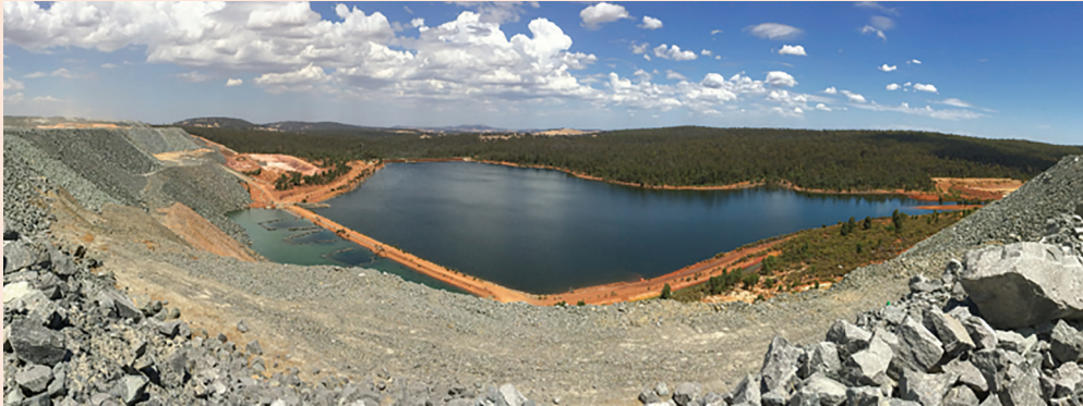
Newmont's Boddington Mine in south-west Western Australia. The mine separates potentially contaminated water drained from the waste dumps from the raw water storage facility in the background. The water is pumped back to the plant to be used preferentially in place of raw water.
