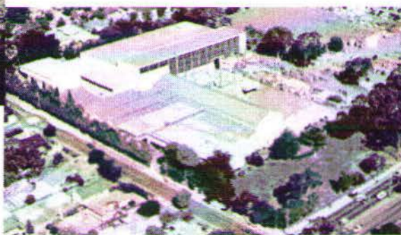
Glen Waverley power transformer plant
