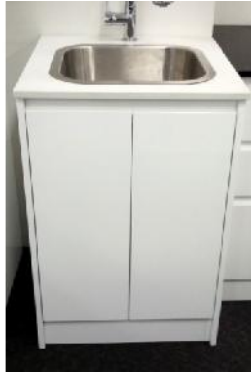
Image 2: A laundry tub bowl fitted on top of a laundry cabinet (Dimensions: 590mm (W) x 580mm(D) x 880mm(H)) (Source: ATTACHMENT D )
