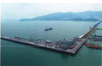
Vale Jetty, Sri Manjung
