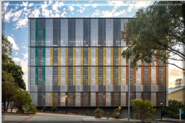
ECU Science Building, Joondalup WA Capral sheet used on periodic table facade
