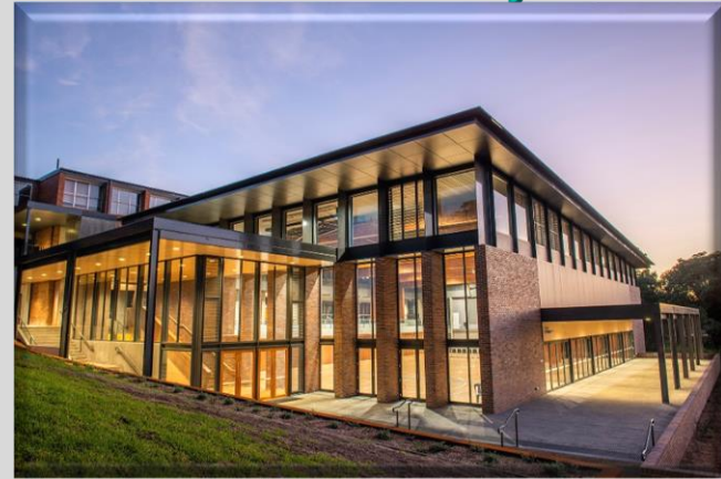
San Clemente High School, Mayfield NSW Won the Master Builders Association Newcastle Excellence in Building Award
