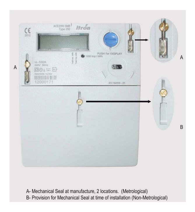
Itron Model ACE2000 Type 292 Electricity Meter (including sample markings and typical sealing)
