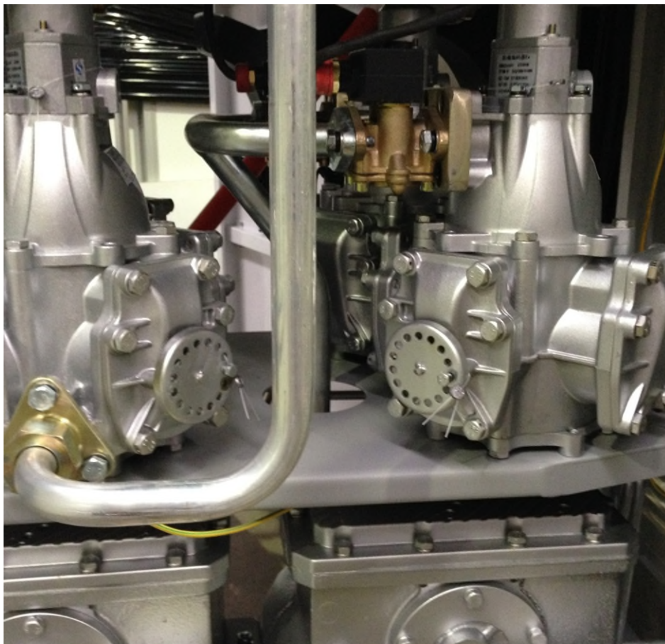
Beijing Sanki Petroleum Technology Model FM-500 Flowmeters
