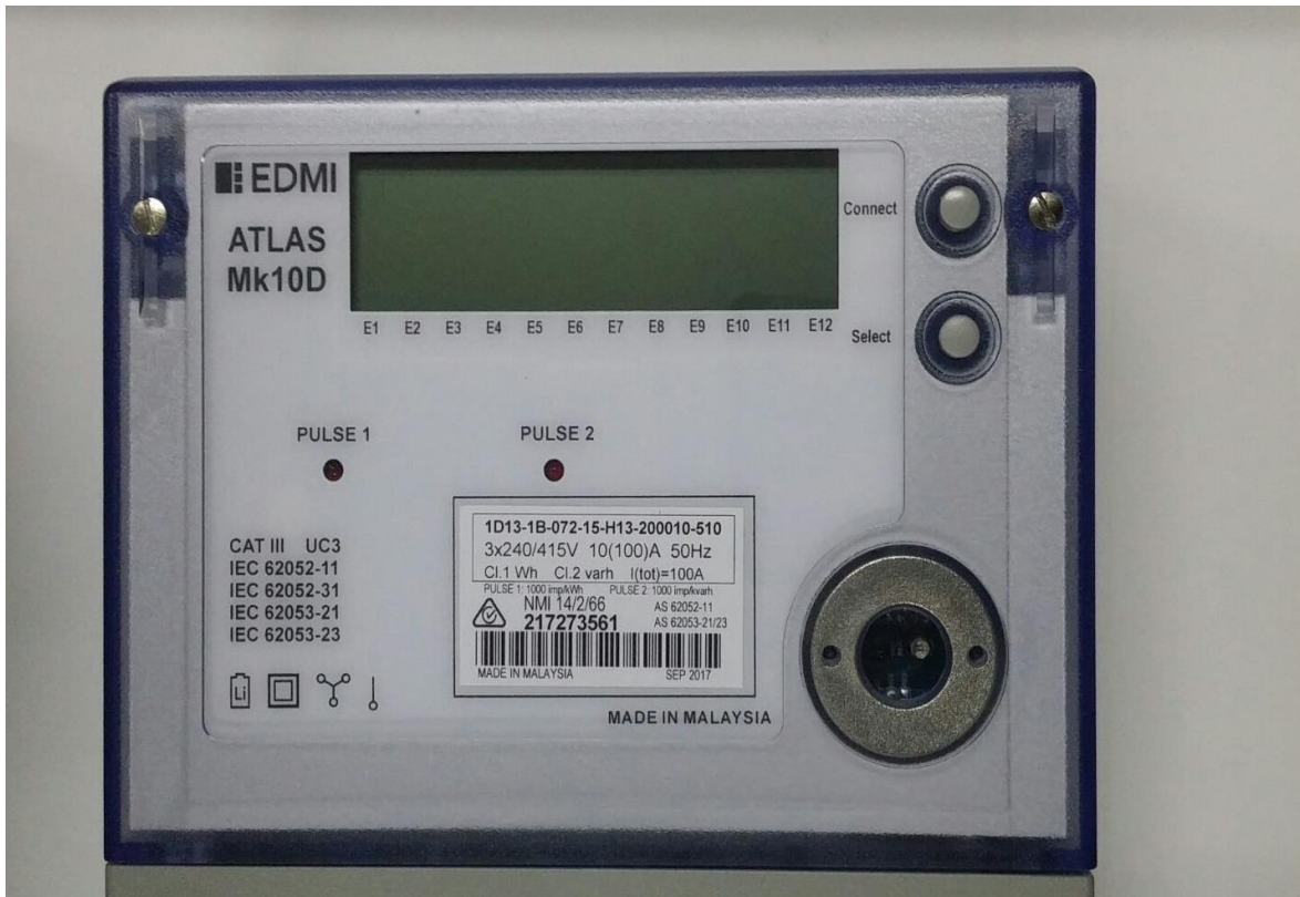
Variant 1 of EDM I Model Mk10D Class 1 Electricity Meter showing the manufacturing code '1D13'
