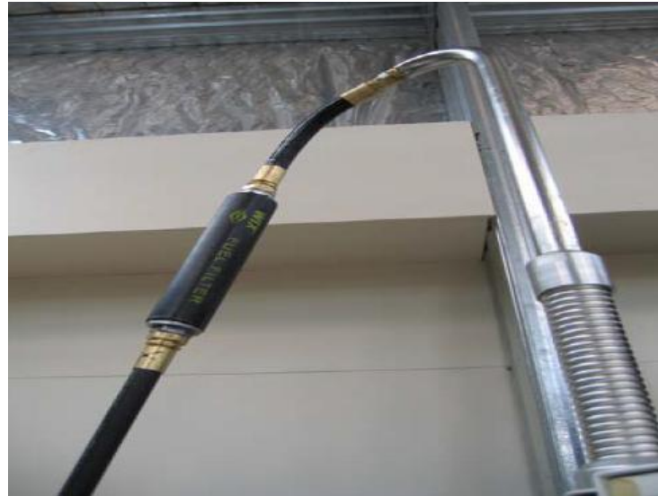
Typical External Filter Installation – Variant 10
