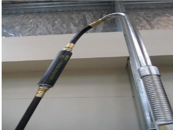
Typical External Filter Installation – Variant 10
