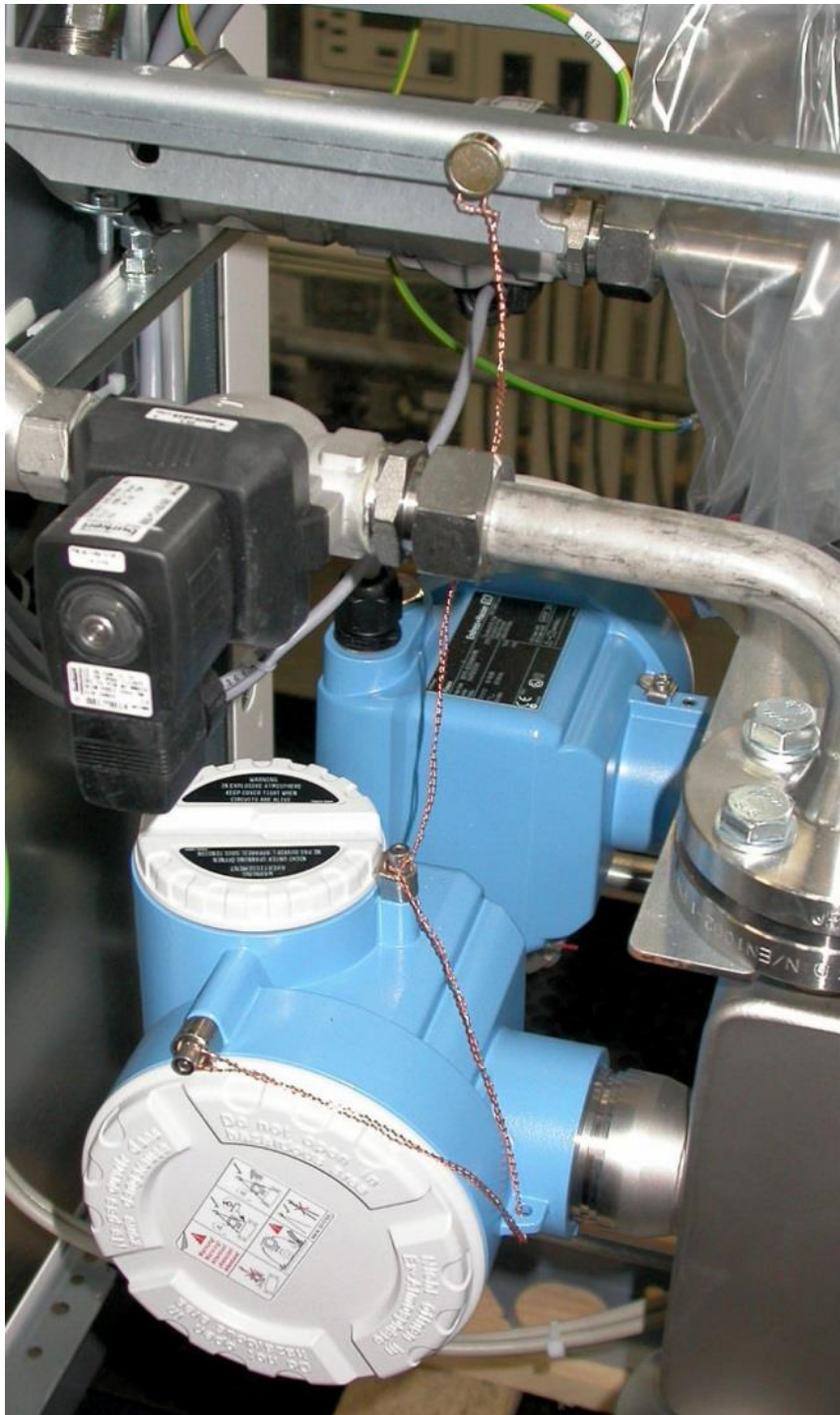
Typical Sealing of Coriolis Meter Calibration Access Including ModBus Connections (Variant 4)
