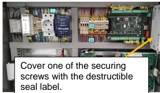
(a) Sealing Location of DIBAL LS-4000, LS-4500, and CLS-4500
