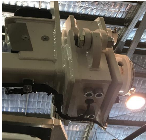
(b) Load Cell Installation
