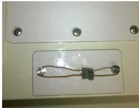
(a) Lead and Wire Type Sealing Arrangement
