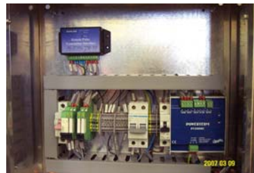
Typical Banlaw FuelTrack Control Box
